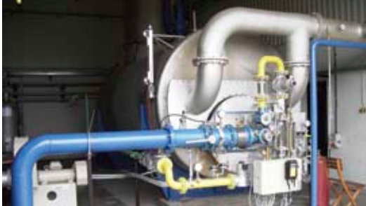
Stainless steel reboiler with special burner for natural gas (System BUSE ERZ 0500)
